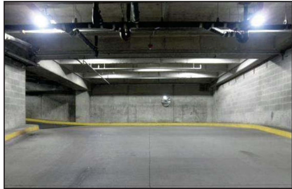
After: (7) 49w LED fixtures
